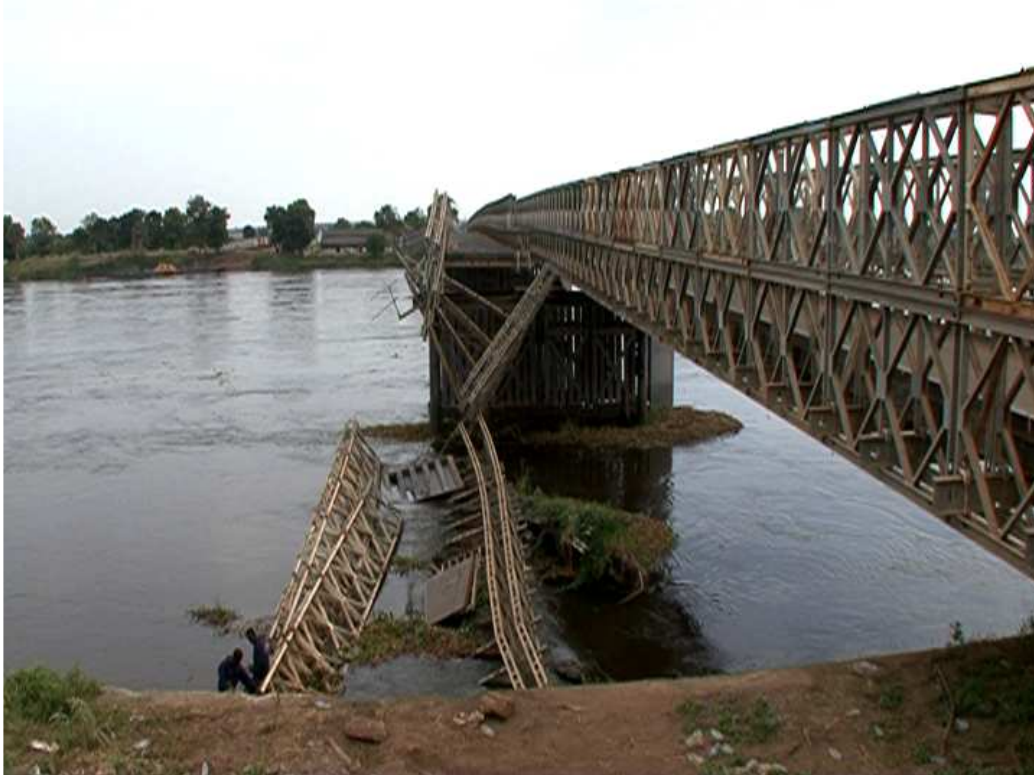
Picture 30: Bridge over the Nile, Juba
