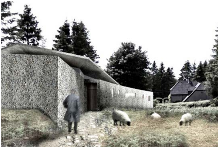
Fig. 8 Detail showing granite aggregate. Image courtesy of David Sheppard
