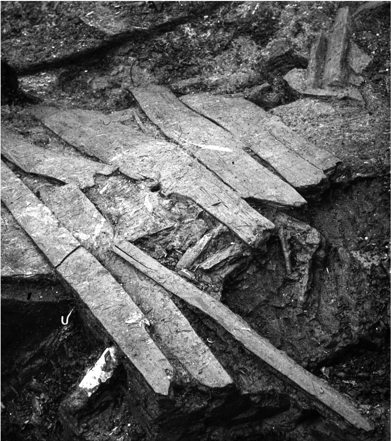
Figure 8.6 Bergschenhoek, a platform of planks (National Museum of Antiquities, see also appendix V).
