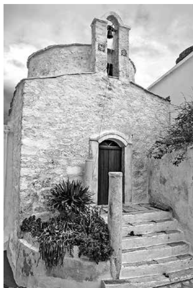
Fig. C.42: C28, view of the church from the west.
