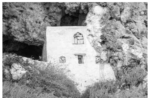
Fig. C.19: C12, view of the church from the east.
