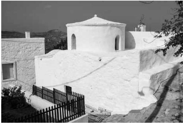
Fig. C.52: C33, view of the church from the south-east.
