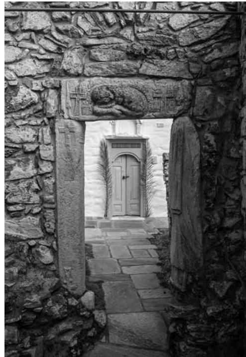
Fig. C.93: C55, the internal gate of the monastery courtyard; the lintel and the post on the left are products of the Ottoman period; the right post is part of an ancient statue.
