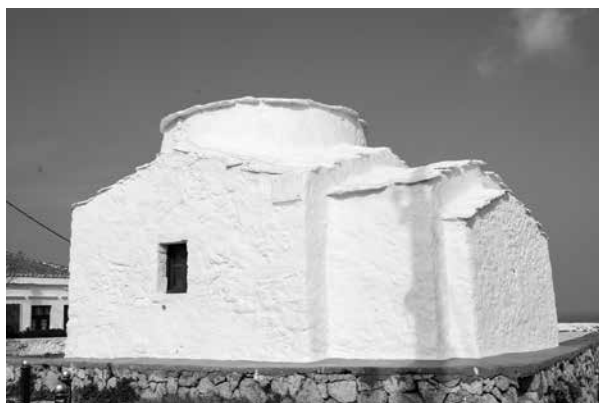
Fig. C.21: C16, view of the church south-east.
