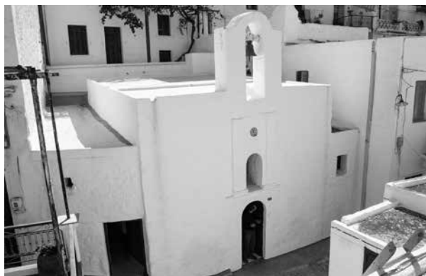
Fig. C.57: C35, view of the church from the west.
