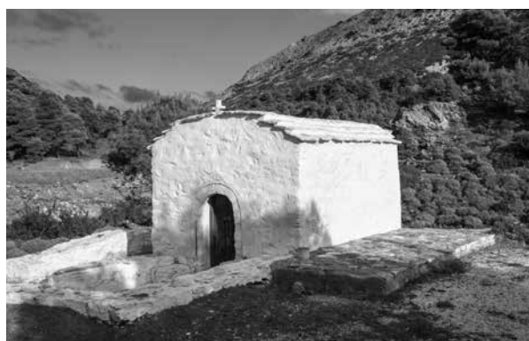
Fig. C.95: C56, view of the church from the south-west.
