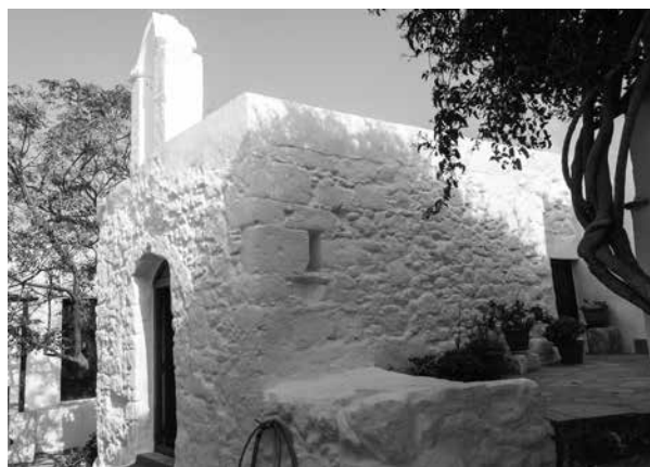
Fig. C.47: C30b, view of the church from the north-west.
