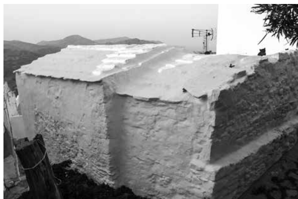
Fig. C.55: C34a, view of the church from the west.
