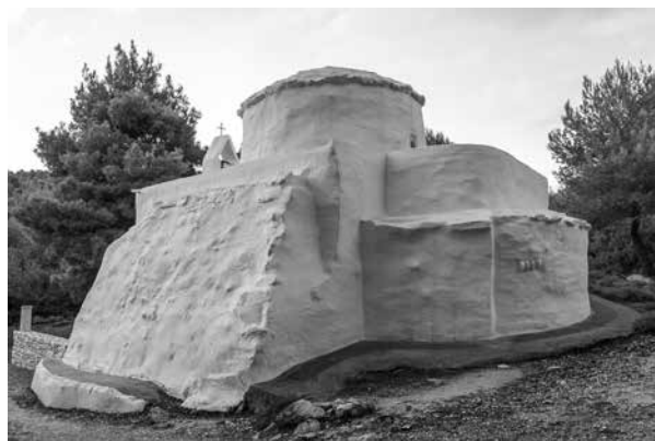
Fig. C.88: C54, view of the church from the south-east.
