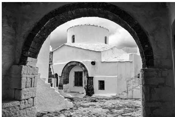
Fig. C.29: C23, view of the church from the north.
