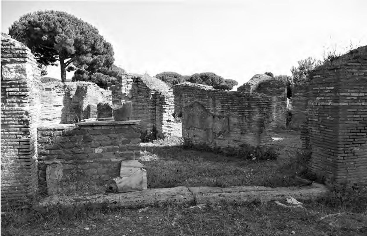
Fig. 7.1 Taberna in the north-east corner of building I XII 10, belonging to the Terme del Foro. (Photo: M. Flohr)
