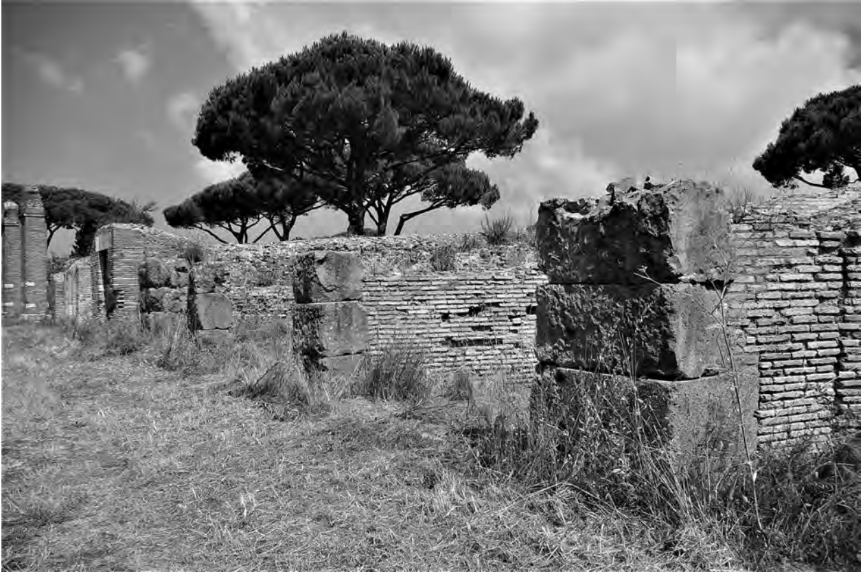
Fig. 7.5 Ostia, ashlar façade of building I XIII 3. (Photo: M. Flohr)
