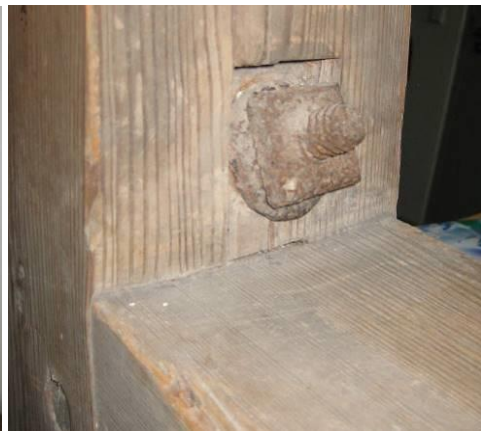
Moerbout in spantbeen
