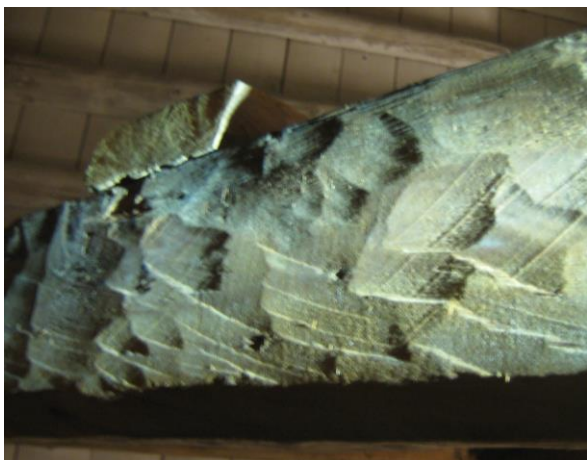
88 Haksporen Lammermarkt 57, direct na 1611
