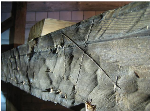
87 Haksporen Lammermarkt 57, direct na 1611
