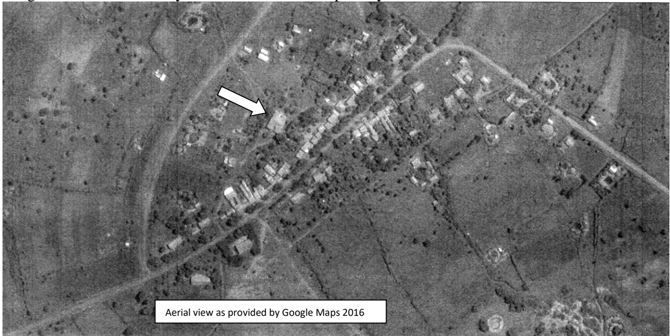
Image 2. Aerial View of Nyamburi Central and Dispensary.
