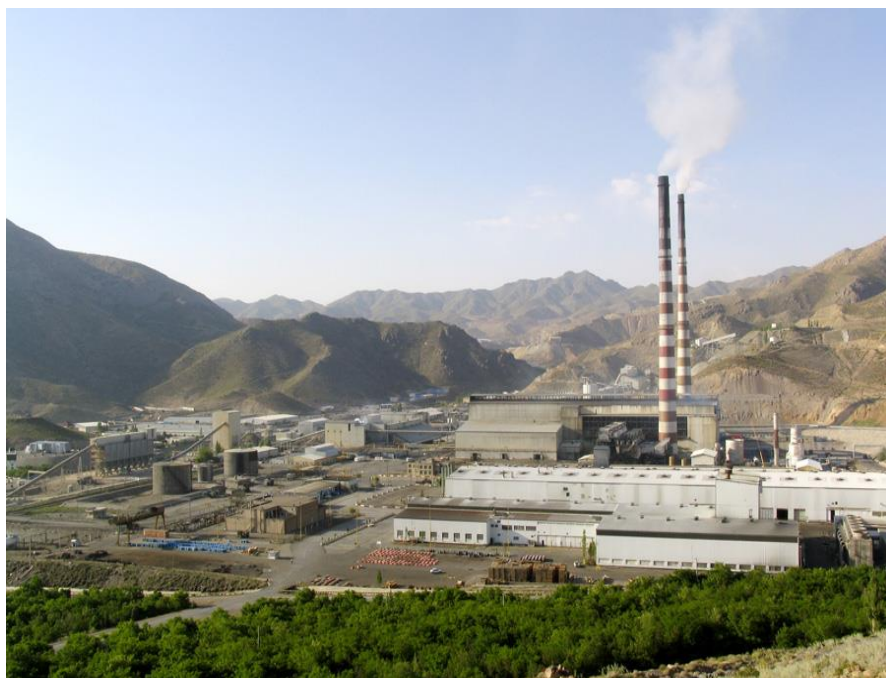
Figure 1: Sarcheshmeh Copper Complex (Image courtesy of NICICO)
