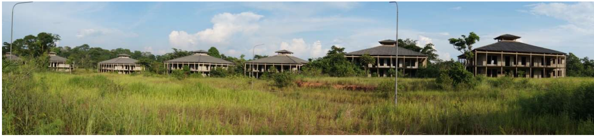
Figure 41 Pan-African University of Libenge View of the students' dorms (11 in total) of the Pan-African University. Notice the lampless electricity poles (Photograph by Mirjam de Bruijn, Libenge 11 June 2014)
