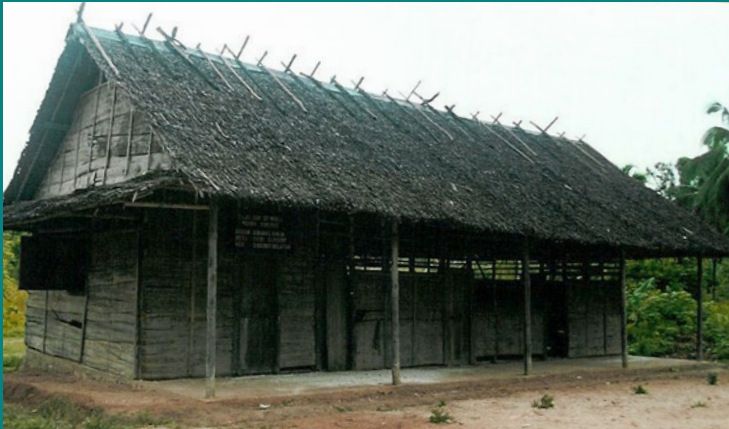
School building in Labongkurong and governmental primary school in Muara Saibi, Siberut.
