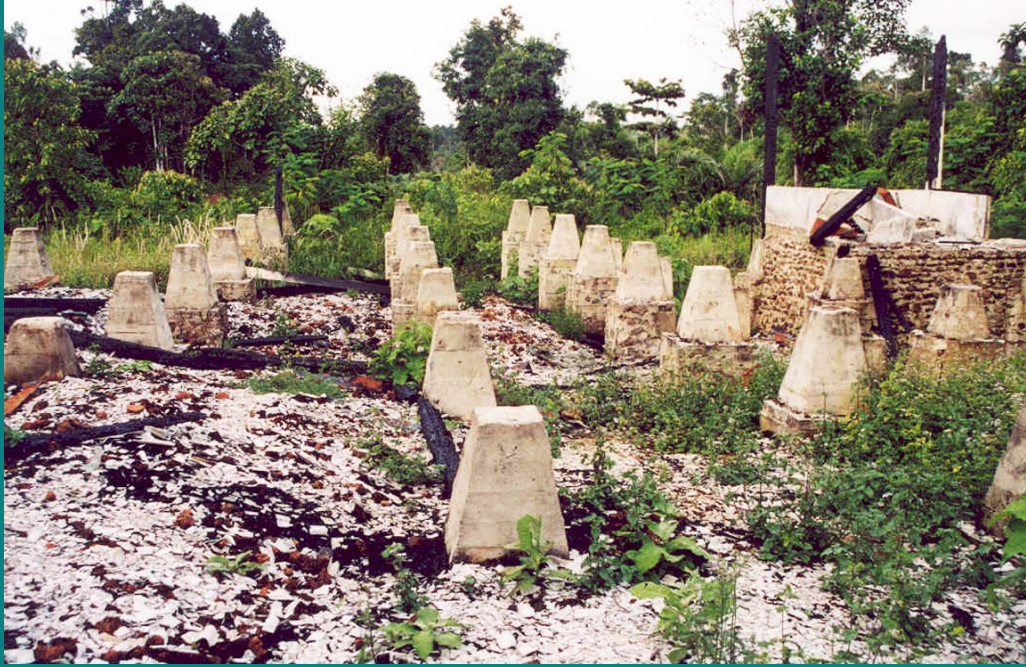
The burned down DPRD office under construction
