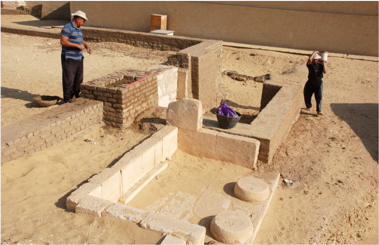
Fig. 33: Strengthening and capping of the outer wall of the tomb of Ry in the southern part of the Dutch-Italian concession. Photo by Nicholas Warner/Leiden-Turin Expedition to Saqqara.
