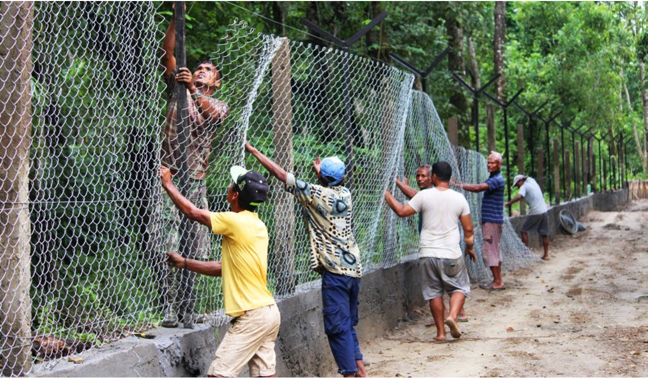
Figure 6.1 Buffer zone users erecting of a wire mesh fence along the forest settlement border to stop animals entering agriculture fields and settlements. Various kinds of fences installed along the forest edges have contributed to reducing the negative wildlife impacts on humans.
