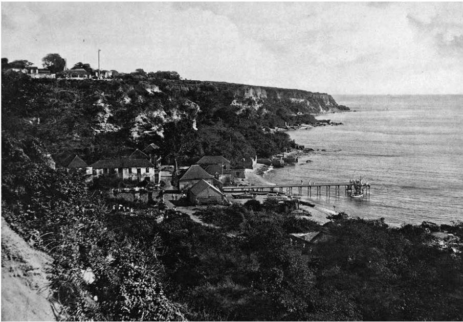
Figure 4.17 The pier and Lower Town in 1910 or shortly after. At this time, the stone docks had already been destroyed by the sea. Source: private collection, St. Eustatius resident.
