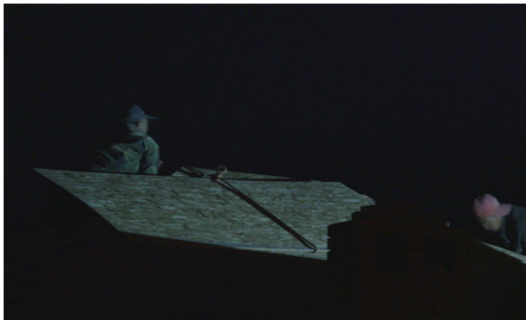
Image 3: North Korean labourers working on a roof (taken from raw footage in Vladivostok).
