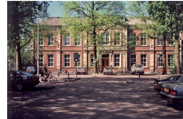
In 1983 CML moves to the building Garenmarkt 1b. Photo CML, 1983
