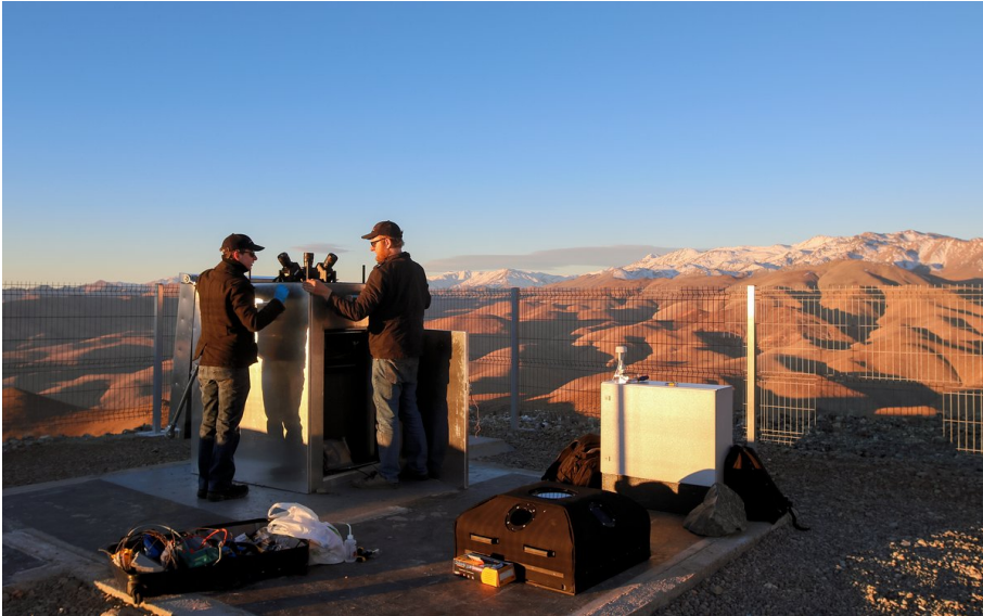
Figure 1.4: The MASCARA station located at La Silla observatory in Chile, shown during the final stages of construction in June 2017. The camera box has been opened so the lenses can be cleaned, allowing the cameras and lenses to be viewed at the top of the instrument. The camera box can be seen at the bottom of the image as the black object with circular windows. The author (right) and Gilles Otten (left) are also visible.
