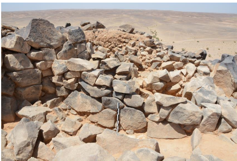
Figure 5.38: Exterior of chamber D, which was constructed against the façade of the main tower of Structure 13 (QUR-2). Scale is 50 cm, photo by P. Akkermans.
