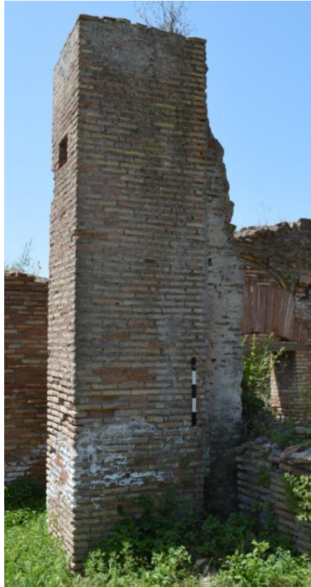
Figure 4.122: The water tower (feature 26) viewed from the north in 2016, with the white coating of calcium carbonate visible on its inner lip.
