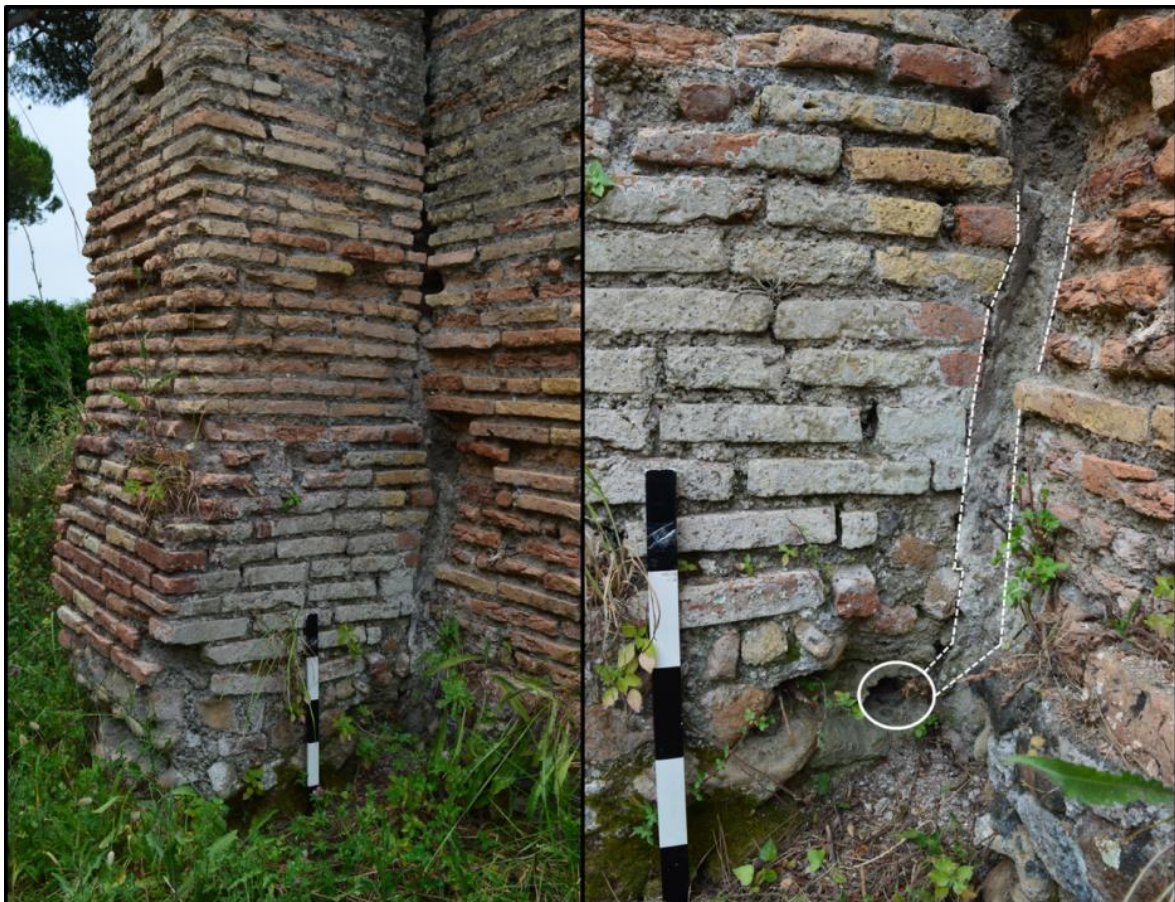
Figure 4.173: View looking south at the pier on the east side of IV, ii, 14. Preserved indentation of lead pipe outlined in dashed lines.
