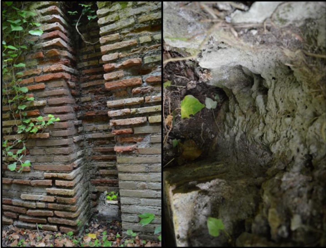
Figure 4.176: Different shaped downshafts in insula IV, ii indicate a division of upper floor waste removal. At right is the semi-circular downshaft in building IV, ii, 9 (feature 61), and at left is the rectangular downshaft from building IV, ii, 13 (feature 60).
