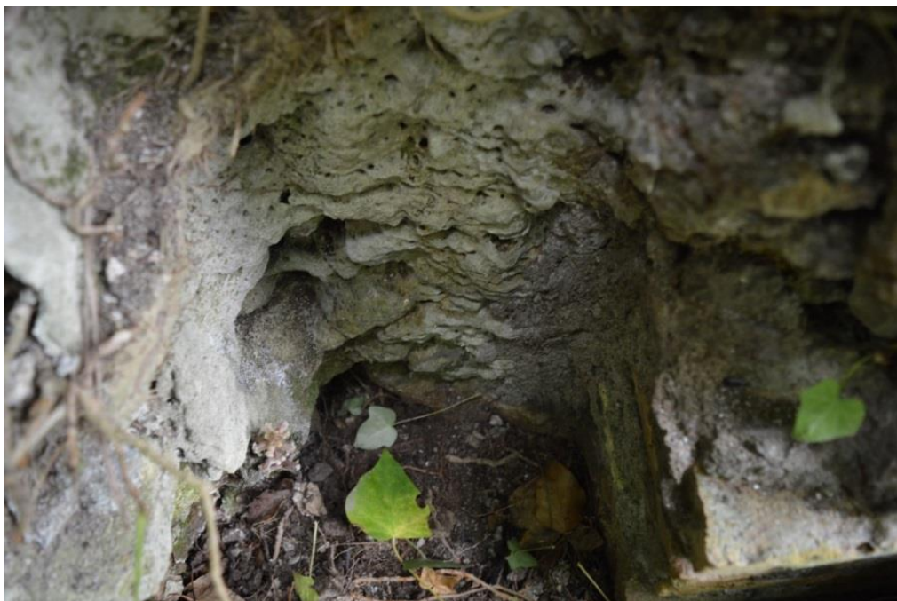
Figure 4.164: View looking down the inner face of feature 61 with the thick and irregular coating of sinter.
