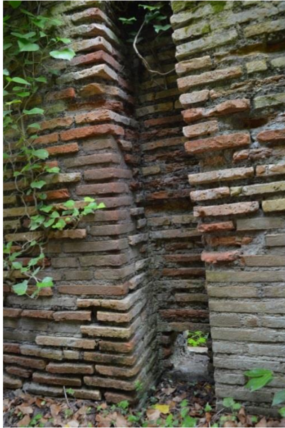
Figure 4.163: Downshaft feature 60 with drain 71 at bottom.
