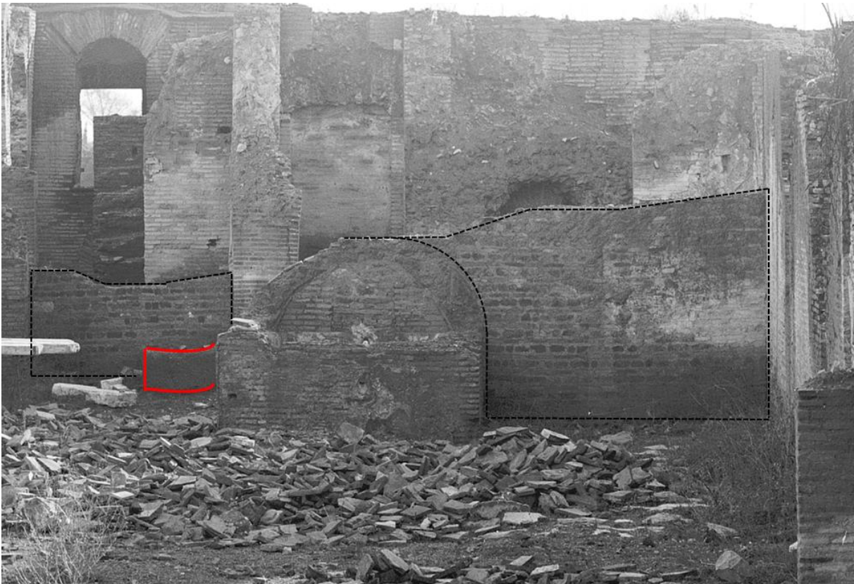
Figure 4.132: Archival photo showing the two walls of opus vittatum outlined in black, the bauletto fountain 68, and the basin 70 outlined in red (SBAO B3036).
