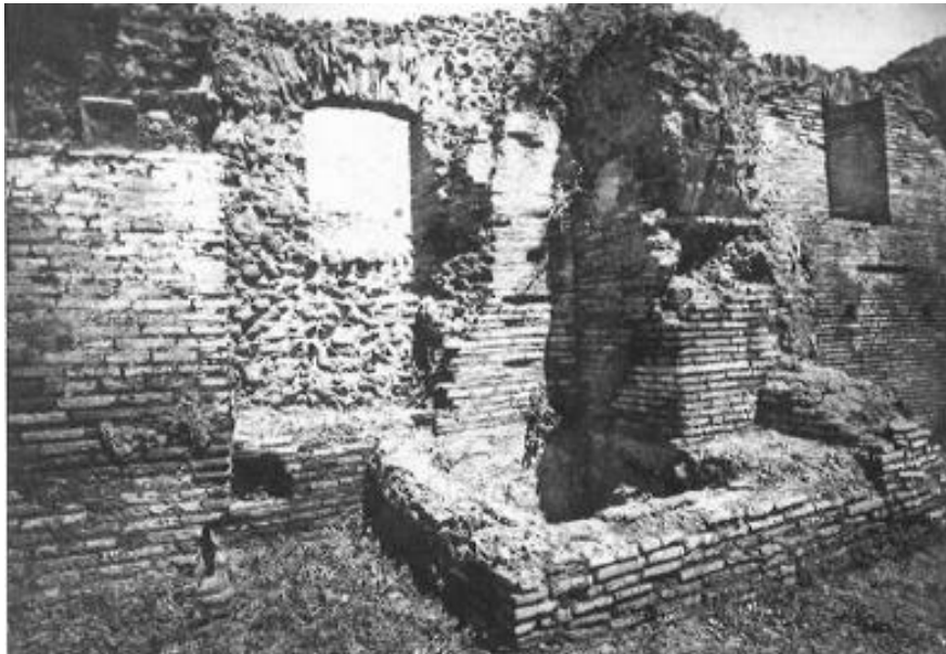
Figure 4.125: North facing view showing basin 30 against the north wall of room 2 before consolidation (RS II, 136, sch. 125).
