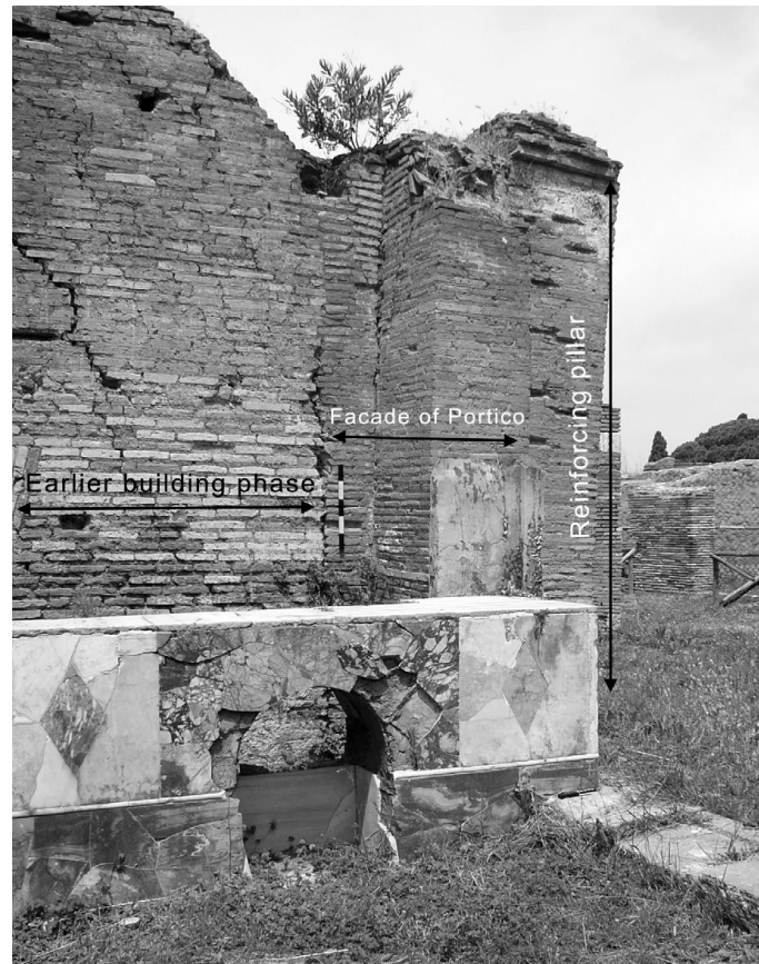
Figure 4.118: Bar counter with its projecting floor level basin, feature 88, (Stöger 2011, 88, Fig. 5.29).
