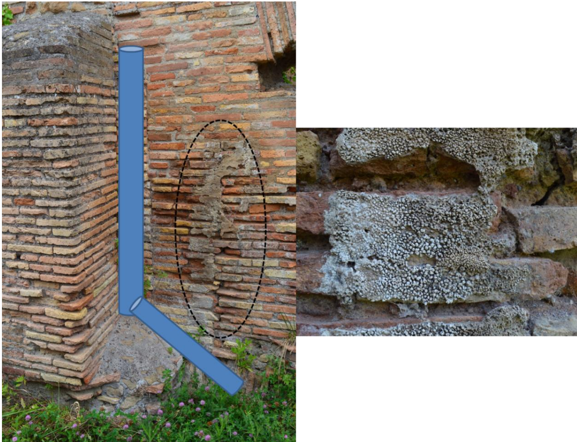
Figure 4.130: West wall of IV, ii, 5, room 09 with calcium carbonate concentration (feature 37). Cylinders indicate possible location of now-lost vertical pipes .
