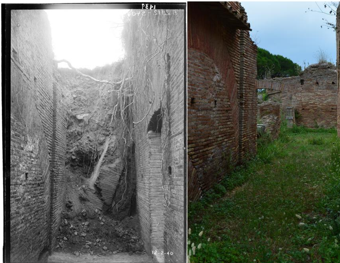
Figure 4.110: The original height of the soil during excavations in 1940 (SBAO B.2912) at left, compared with the current state of the insula at right. Looking south down hallway 20 of the Caseggiato dell'Ercole (IV, ii, 2-3).
