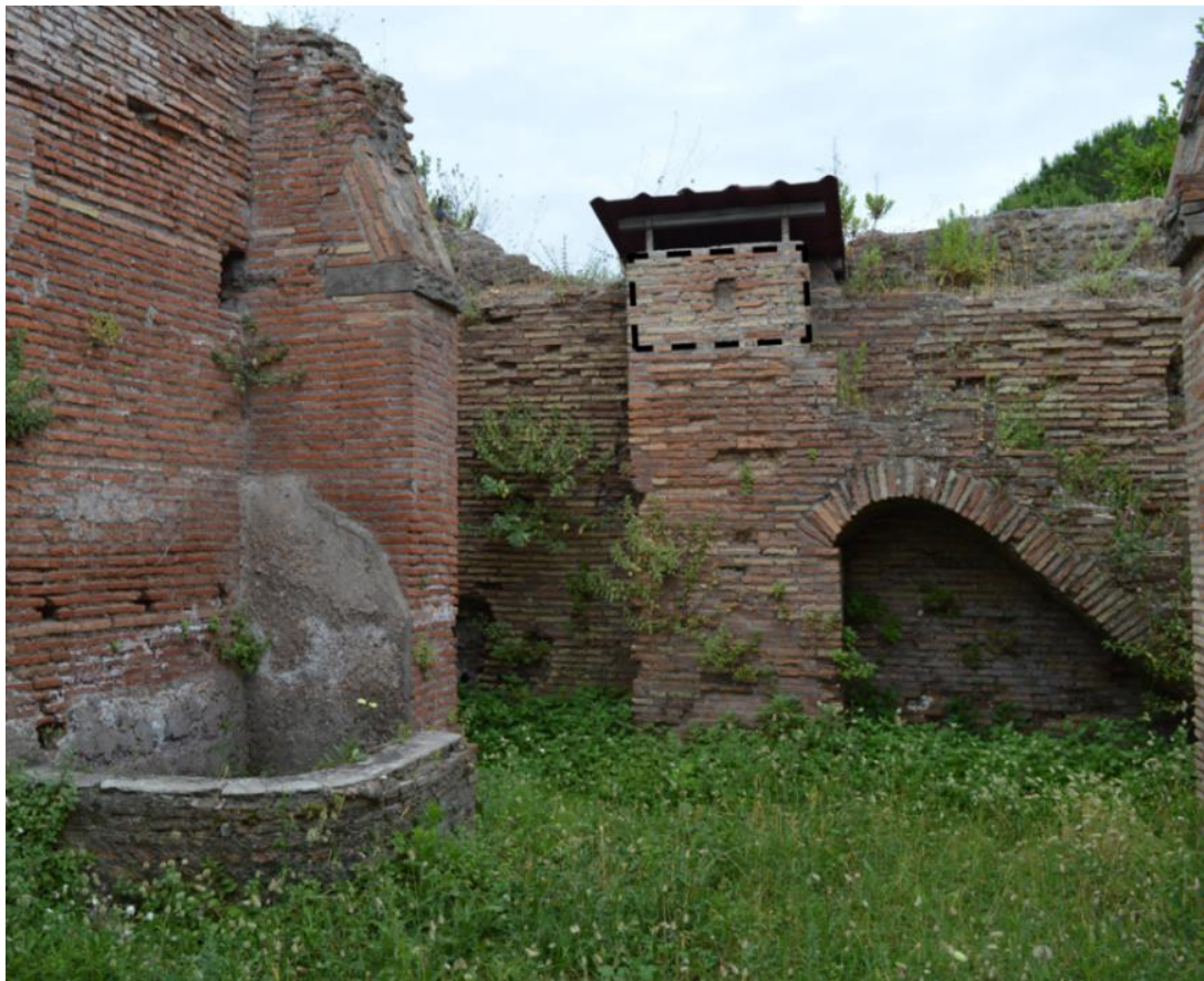
Figure 4.179: Looking south at the flight of stairs leading to the top of the cistern, with the distribution basin indicated by dashed lines.
