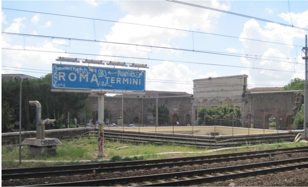
Figure 2.18: The Porta Maggiore in Rome, seen from the Roma Termini train station with two superimposed aqueduct channels to ensure that the different types of water remained separated from each other.
