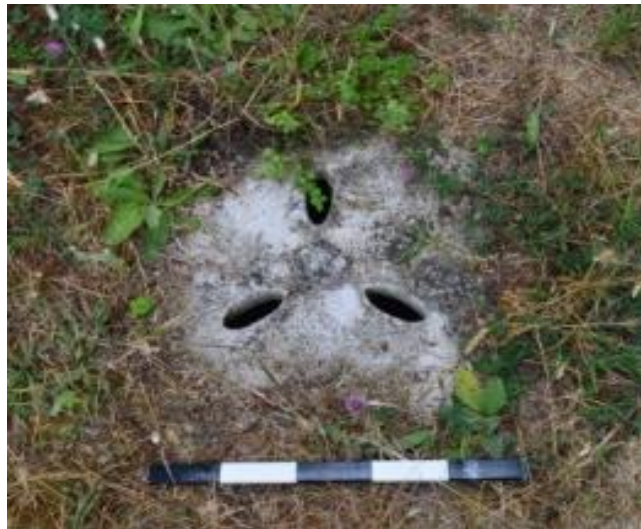
Figure 1.12: Example of a man-hole cover at Ostia (in IV, ii, 1), with its lozenge shaped openings of ca. 3 x 10 cm.
