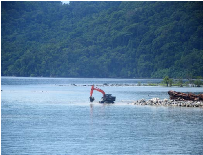
Plate 21. Excavator making wharf at Ruarata, East Are'Are 2017.
