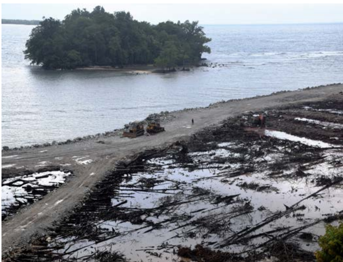
Plate 22. Removal of mangroves for log pond construction at Ruarata, East Are'Are 2017.
