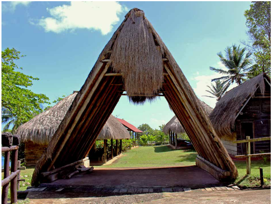
Figure 14: Entry to the Kalinago Barana Autê, Dominica.
