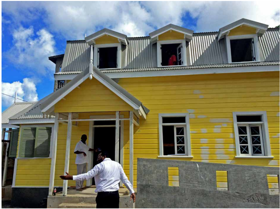
Figure 57: Walcott Place, St. Lucia, while under construction in October 2015.
