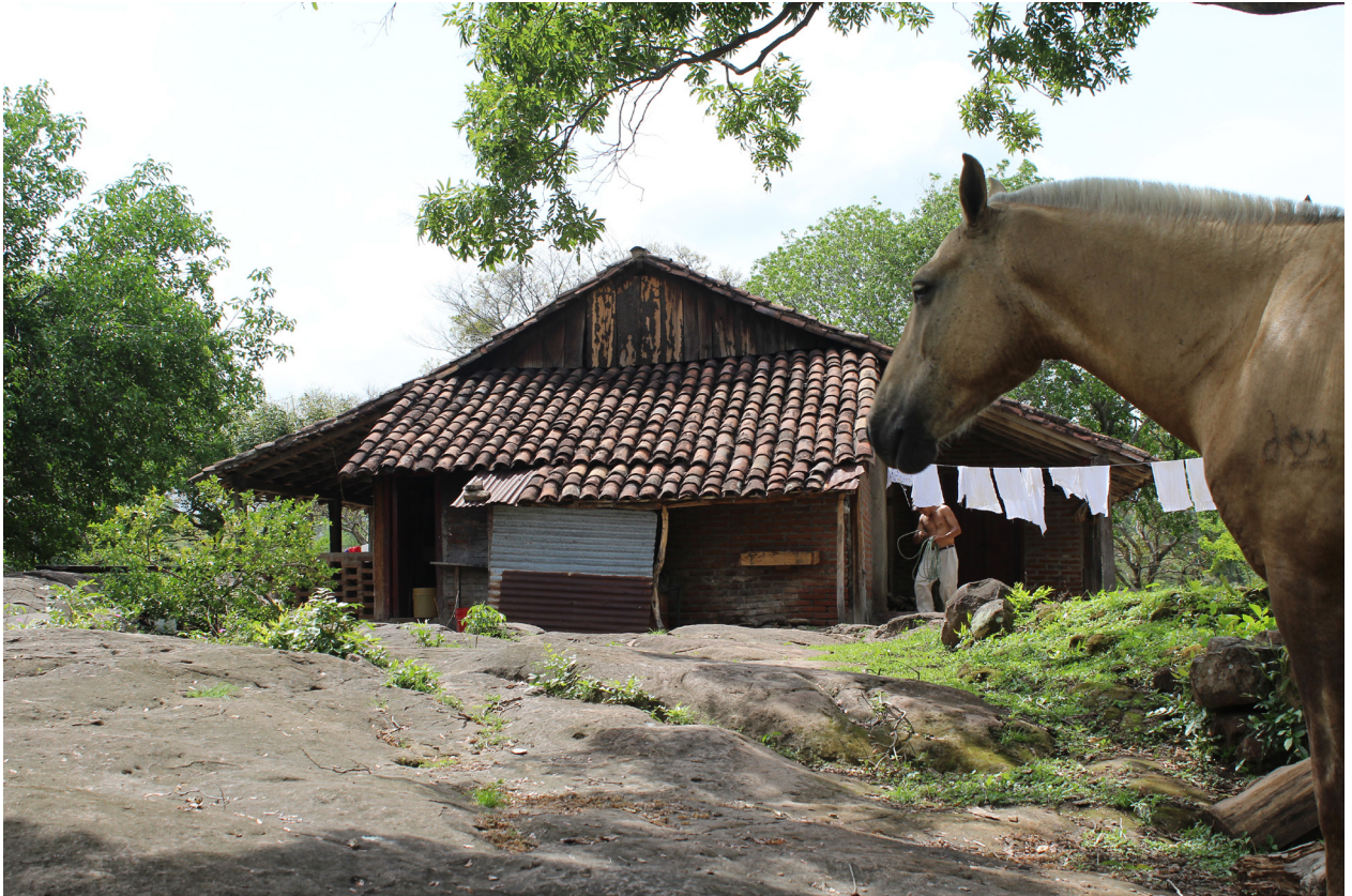
Figure 225: Example of a contemporary house in the area, for which bedrock was used as a foundation (credit: Alejandro Arteaga).
