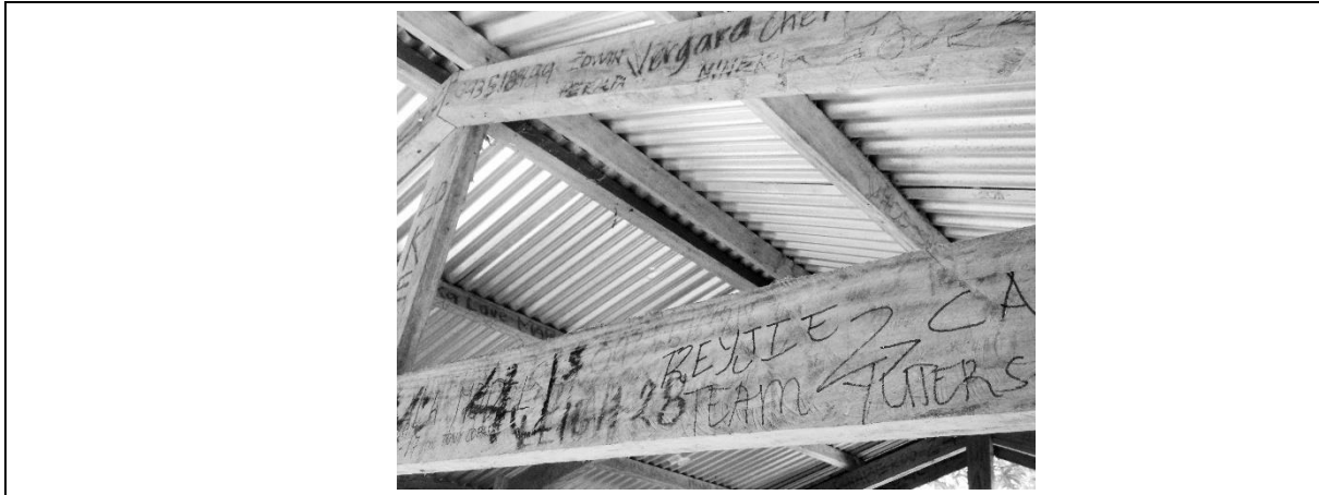
Photo 4: Vandalism in Duba Cave (Photo by L Righetti 2018)
