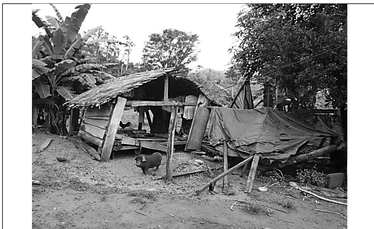
Photo 1: A house categorized as totally damaged (Photo by J Janson 2019)
