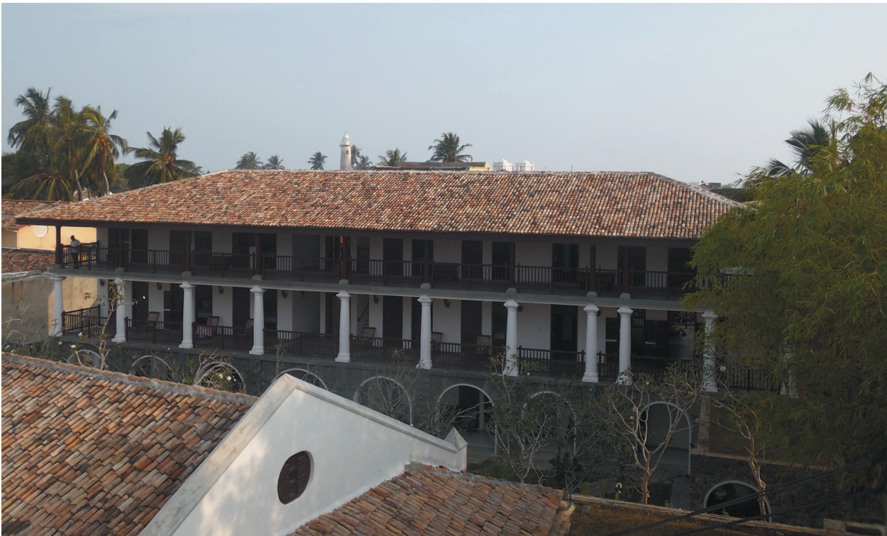
Fig. 272 The same building after the completion of the work in 2018.
