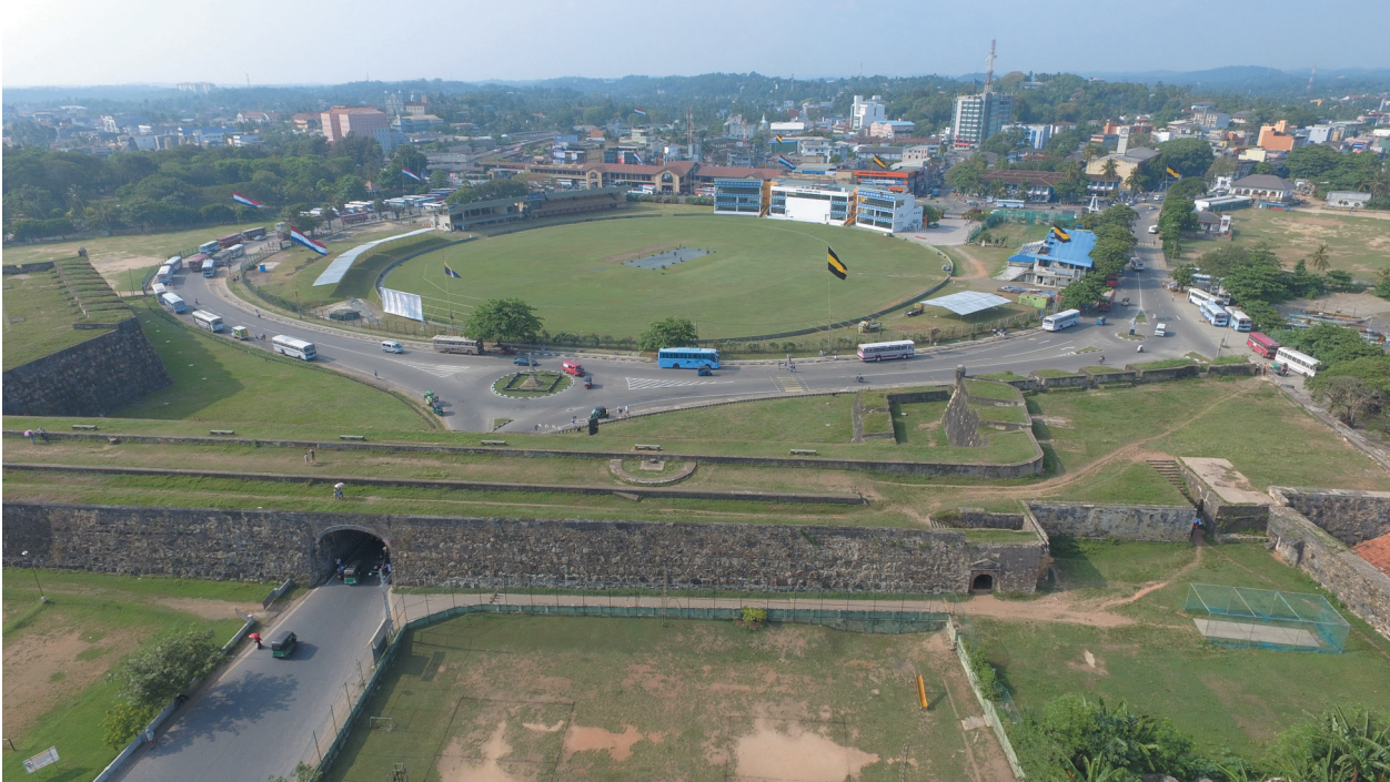
Fig. 277 The stadium (2016) with the new pavilion to the north.
