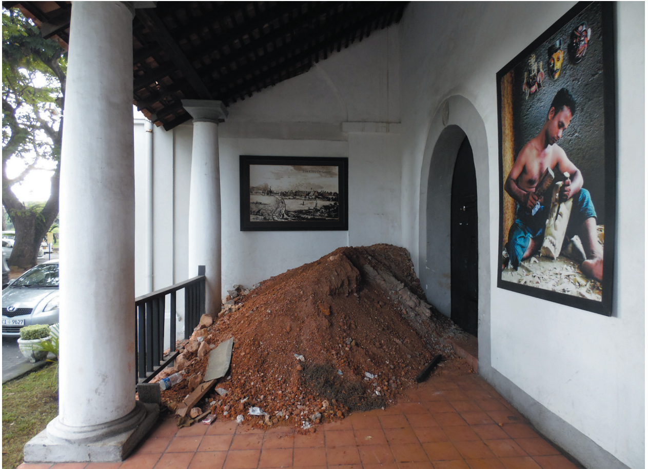
Fig. 273 Excavated pile of earth on the verandah (November 2015).
