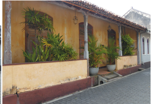
Figs. 228–229 Prominence of restored architecture: a foreign-owned property during (2016) and after restoration (2017).
