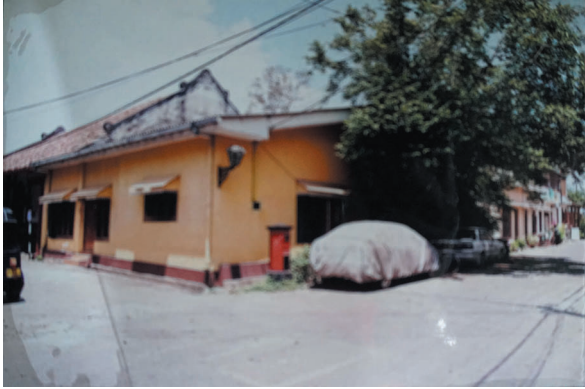
Fig. 259 The house after renovation in 1998 (image courtesy of Mr Rathna Sri Wijesinghe).
