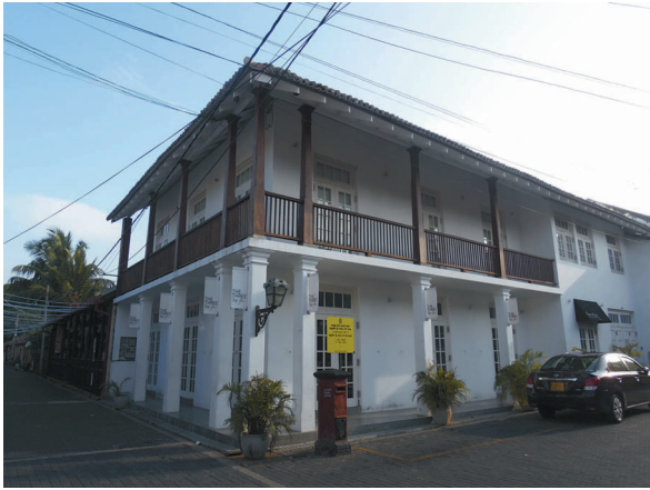
Fig. 260 The building in 2016, after renovation by the foreign owner. The red postbox in the middle of the image is the only visible feature from the 1990s.
