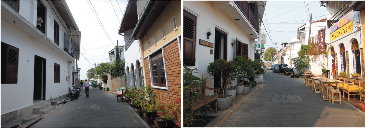
Figs. 188–189 Streetscape of a formerly residential street in March 2016 (left) and in January 2018 (right). The formally residential buildings to the left and right have respectively changed into a tourist accommodation and a modest family-run restaurant.
