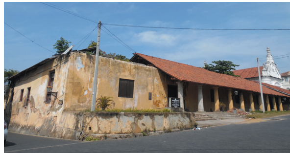
Fig. 95 The same building in 2018 with a verandah added in the early ’90s.
