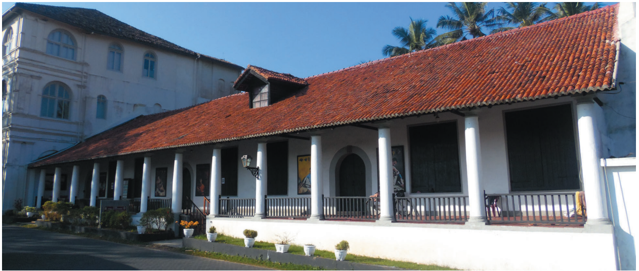
Fig. 97 The same building in 2016, with a full verandah added in the early '90s.
