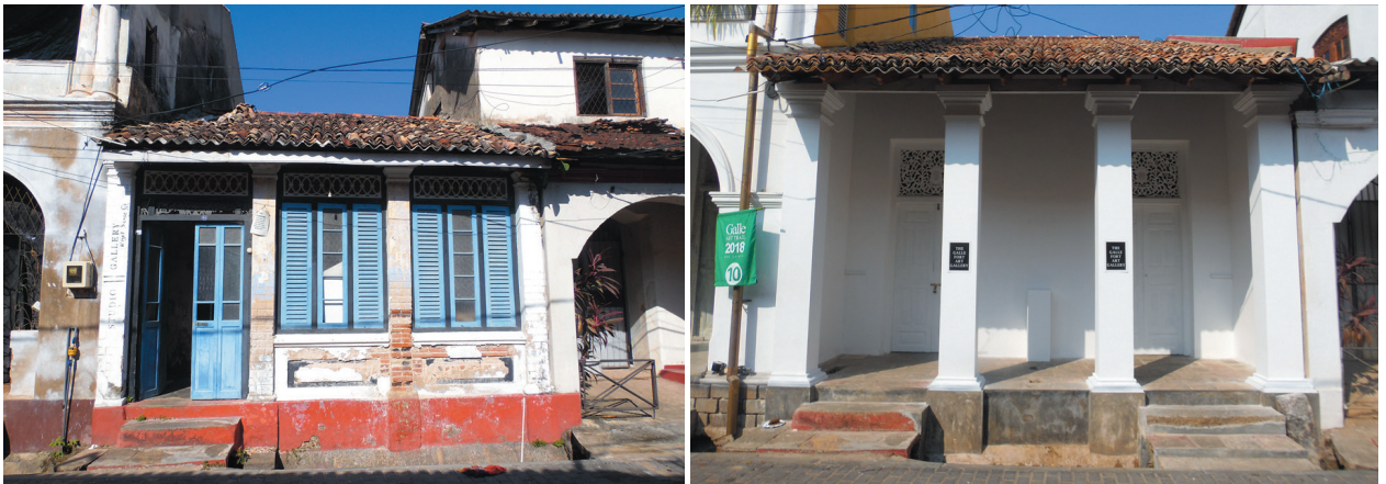
Figs. 184–185 A building in 2016 (left) and same one, in January 2018, as a gallery, after its development (right).
