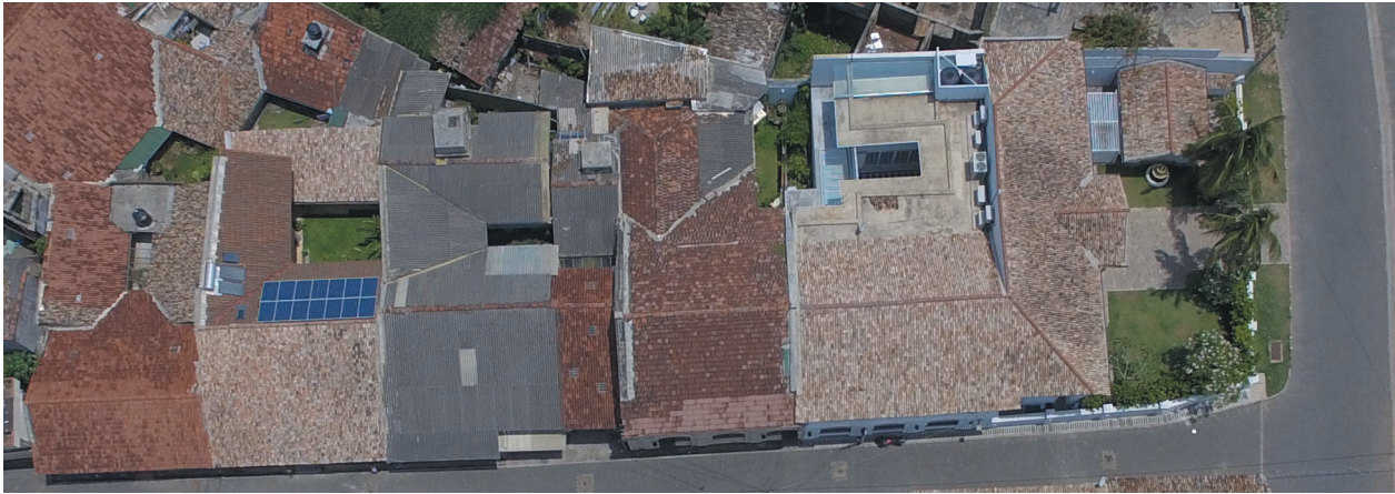
Fig. 133 Roofscapes of the same buildings in 2016: four of them are covered in clay tiles, while only one (in the middle) has the prohibited asbestos. Furthermore, approved developments have positively increased the use of half-round tiles over asbestos (extreme right and the second from the left, also with solar panels).
