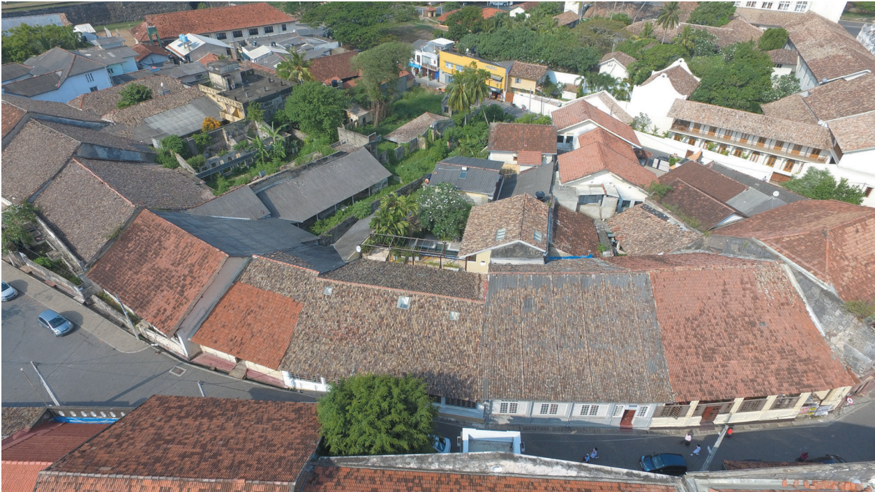
Fig. 47 Aerial view of the streetscape of Middle Street, showing the narrow street frontages and deep interiors of houses.
