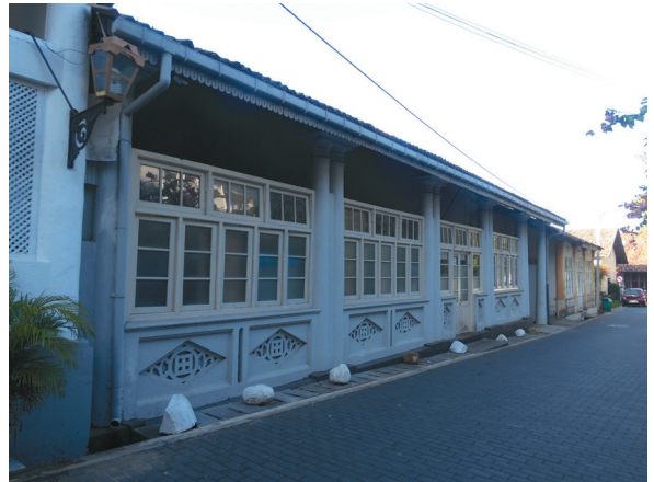
Figs. 55–56 Renovated arched verandahs (above) and a verandah half-covered by glass windows (below).
