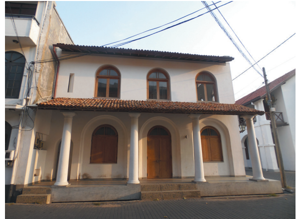
Figs. 82–83 A “disturbing” façade (at left; Kuruppu and Wijesuriya 1992, 145) that changed into a “contributing” façade after an approved development (at right, 2016). 373
