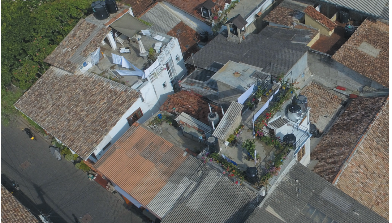
Fig. 168 Rooftops of B&Bs, examples of further vertical constructions halted by the heritage authorities.
