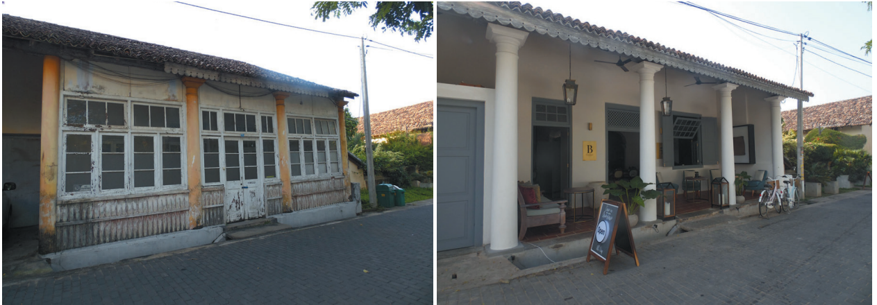
Figs. 182–183 A dilapidated building in 2016 (left) and same as a restaurant in January 2019, after its development (right).
