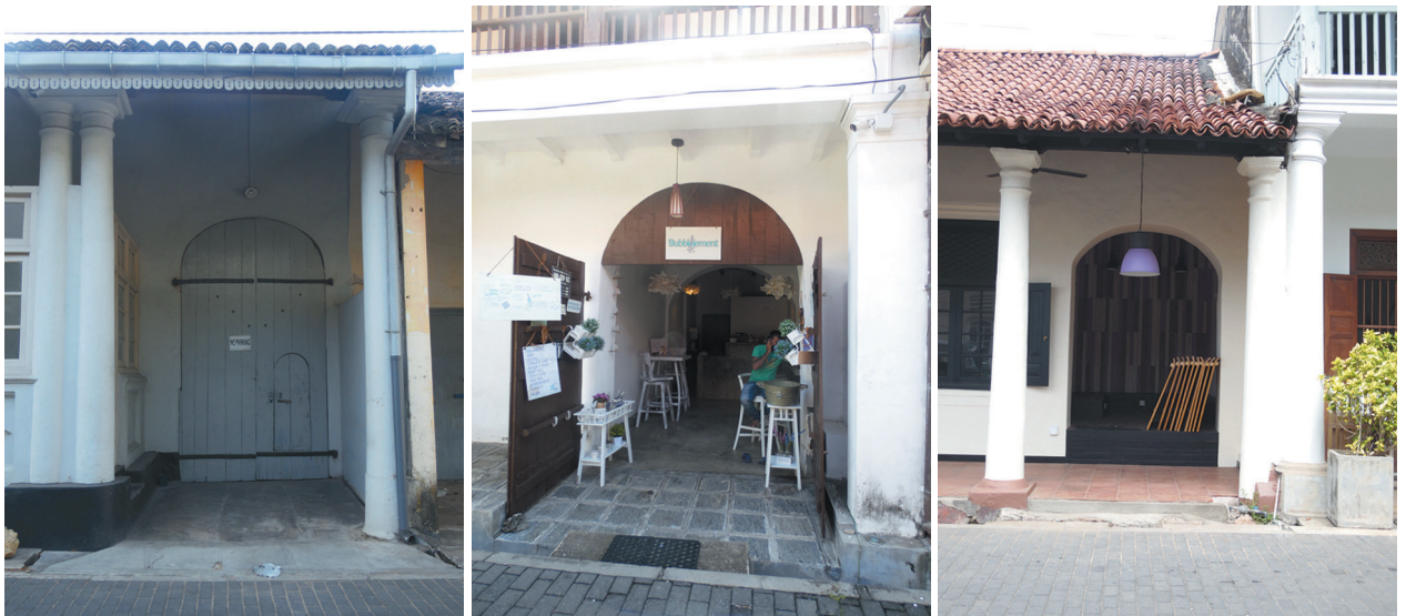
Figs. 136–138 Three stables in different conditions: unchanged (the first one, on Church Cross Street); renovated with positive changes (the second, on Parawa Street); and an ongoing “unpermitted” change, in December 2017 (the third, on Pedlar Street).
