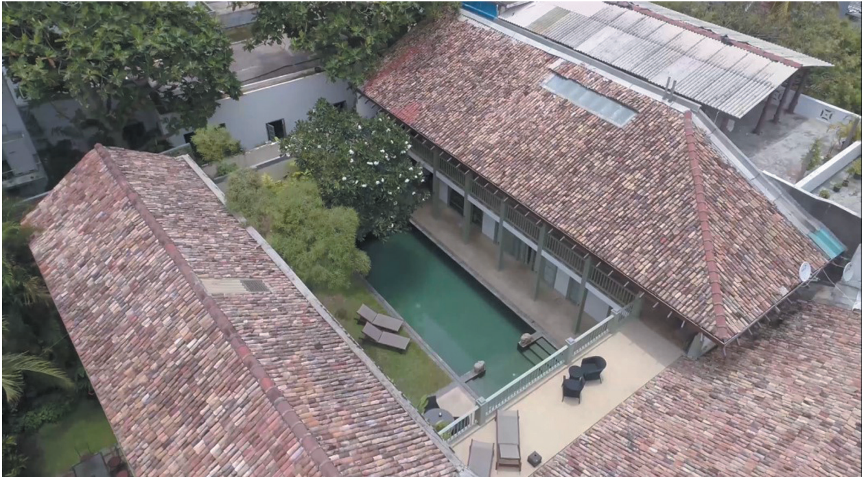
Fig. 178 A swimming pool in a newly developed villa; the pool replaced the former central courtyard. 394
