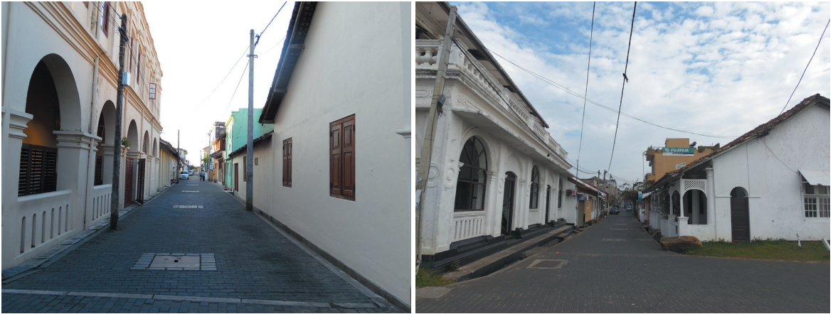
Figs. 125–126 Street views of Church Street with buildings in approved colours, 2016 (the green building in the first image is a mosque).
