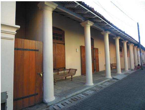
Figs. 53–54 A timber-pillared verandah (above) and a renovated Doric-pillared verandah (below).
