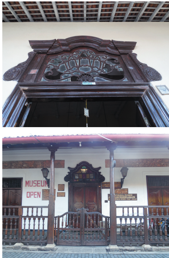
Figs. 51–52 The Dutch-period ornamental fanlights above the doorway at no. 28, Middle Street (above) and no. 35, Leyn Baan Street (below, with a renovated façade).
