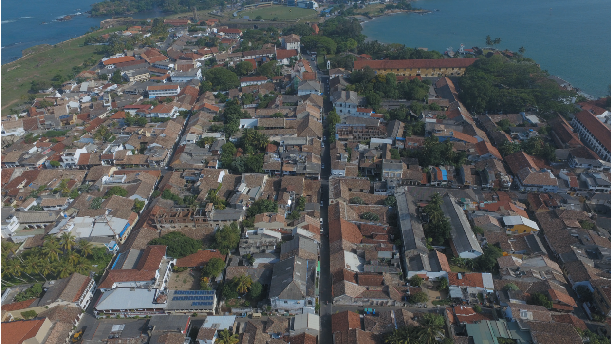
Fig. 135 The roofscapes in 2016, showing more tiled roofs and a substantial amount of prohibited asbestos.
