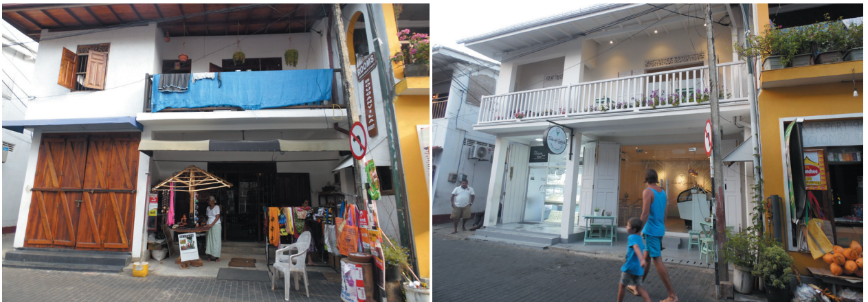
Figs. 186–187 A developed building as a shophouse in 2016 (left) and the same redeveloped with multiple businesses in 2018 (right).
