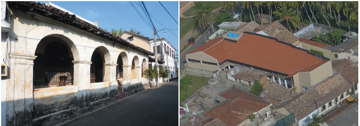
Figs. 143–144 The British façade kept as it is (left) and the aerial view of the development of the same building behind the façade (right), an ongoing approved development of a boutique hotel (2016).
