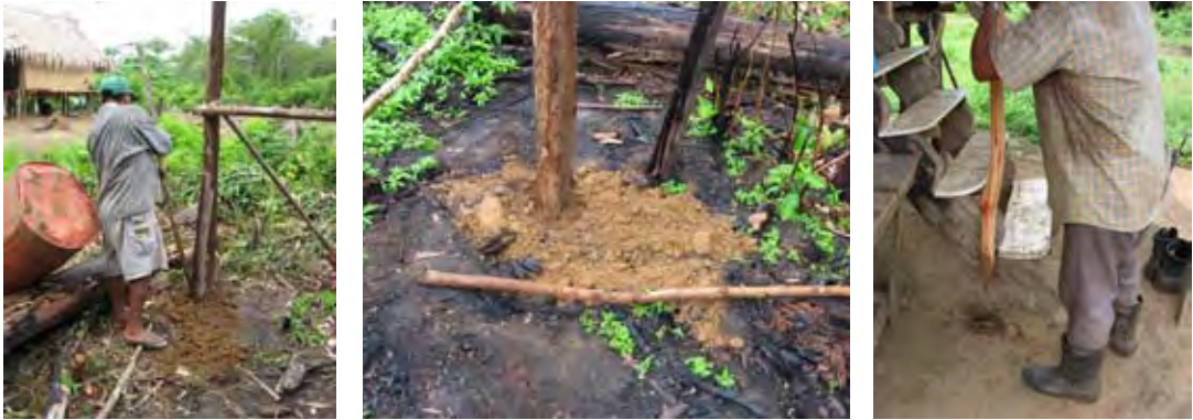
Fig. 3.6: Posts and stakes placed into the soil. L: The posthole with the floor post is filled with soil and pounded with a stick by Paneshi. M: One of the posts with the fresh soil contrasting with the surrounding charcoal soil (due to previous burn clearing). R: Paneshi embeds a pointed stake into the soil by adding water and continuously thrusting.
