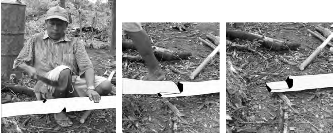
Fig. 3.5: Turning a wakapu post into a support by combining cutting and breaking.
