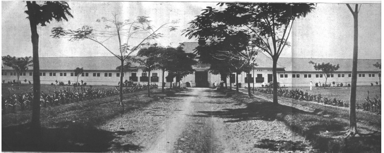
Front view of the state reformatory Tangerang for boys.
