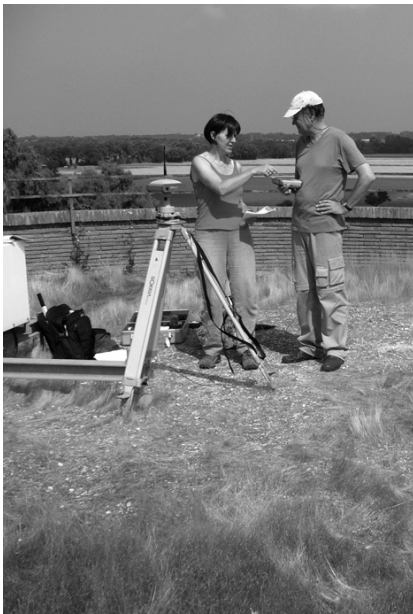
Fig. 4.4 – Setting up the base point on top of the Castello Giulio II
