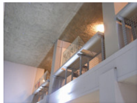
Figure 3.47 Part of the ceiling in the museum. Photo by R. AlGhzawi
