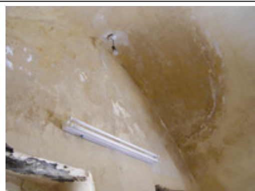
Figure 4.15 Fluorescent and incandescent lamps at the Umm Qeis Museum. Photo by R. AlGhzawi
