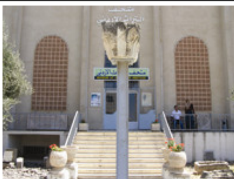
Figure 3.48 The main gate and the stairs. Photo by R. AlGhzawi
