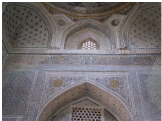
Fig.337: Shahr-i Sabz, Gumbazi-Sayidon, Mausoleum of Ulugh Beg's Descendants, detail of the interior, squinch and arched recess, September 2006 Source: Author's photograph
