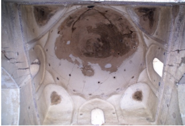
Fig.436: Samarqand, Bībī Khānum Mosque, dome detail with squinches of the southern mosque, September 2006
