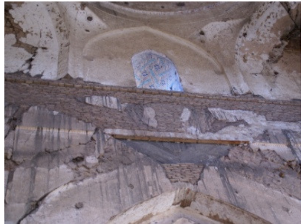
Fig.458: Samarqand, Bībī Khānum Mosque, detail of the damage to the squinches of the dome in the sanctuary, September 2006 Source: Author's photograph
