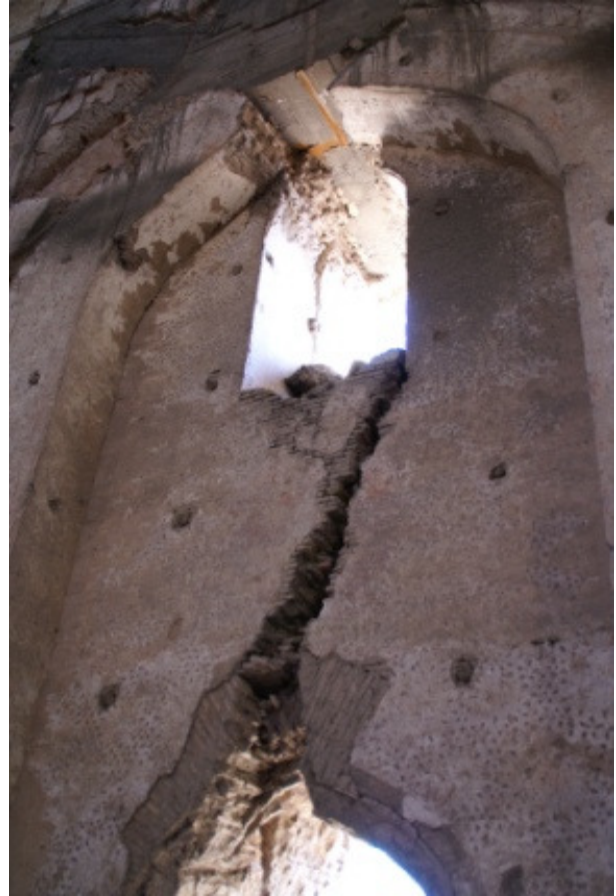
Fig.462: Samarqand, Bībī Khānum Mosque, detail of the damage to the blind niches of the sanctuary, September 2006
