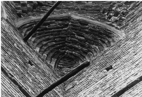
Fig.282: Shahr-i Sabz, Jahangir's tomb, interior detail, brick squinch, 1960 Source: Lisa Golombek, Archnet [Accessed on 1 November 2009]
