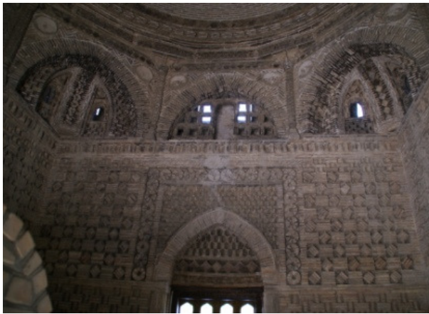
Fig.197: Bukhārā, detail of the dome squinches of the Sāmānid Mausoleum, September 2006 Source: Author's photograph
