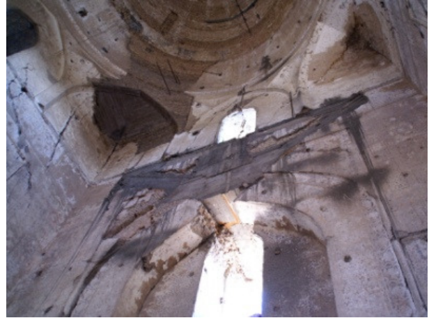
Fig.456: Samarqand, Bībī Khānum Mosque, detail of the squinches of the dome in the sanctuary, September 2006 Source: Author's photograph
