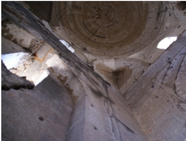
Fig.457: Samarqand, Bībī Khānum Mosque, detail of the squinches of the dome in the sanctuary, September 2006 Source: Author's photograph
