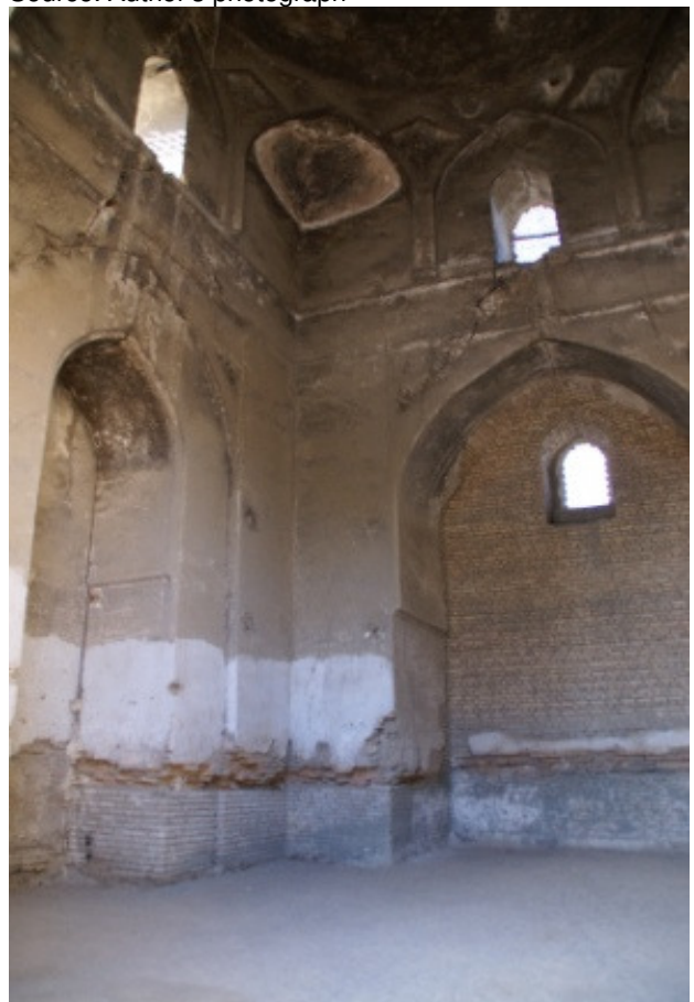
Fig.439: Samarqand, Bībī Khānum Mosque, interior detail with squinches and arched recesses of the northern mosque, September 2006
