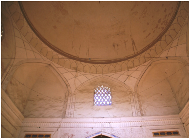
Fig.737: Bukhārā, Nādir Dīvān Beg Khānaqāh , detail of dome with the squinches, September 2006 Source: Author's photograph
