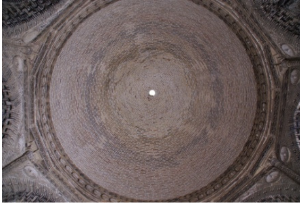
Fig.195: Bukhārā, interior view of the dome of the Sāmānid Mausoleum, September 2006 Source: Author's photograph
