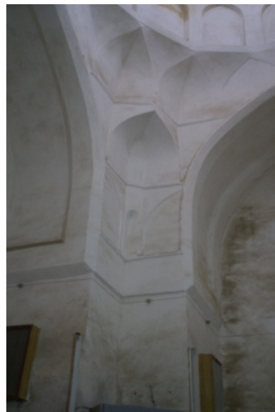
Fig.560: Bukhārā, Ulugh Beg Madrasa, detail of the dome squinches in the south-western chamber, September 2006 Source: Author's photograph
