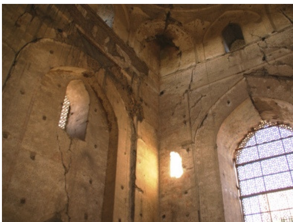
Fig.459: Samarqand, Bībī Khānum Mosque, detail of the damage to the arched niches in the sanctuary, September 2006 Source: Author's photograph
