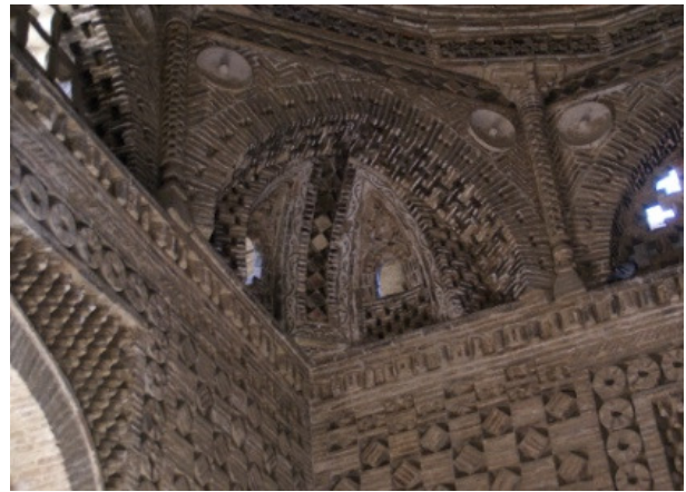
Fig.198: Bukhārā, detail of a corner dome squinch of the Sāmānid Mausoleum, September 2006 Source: Author's photograph
