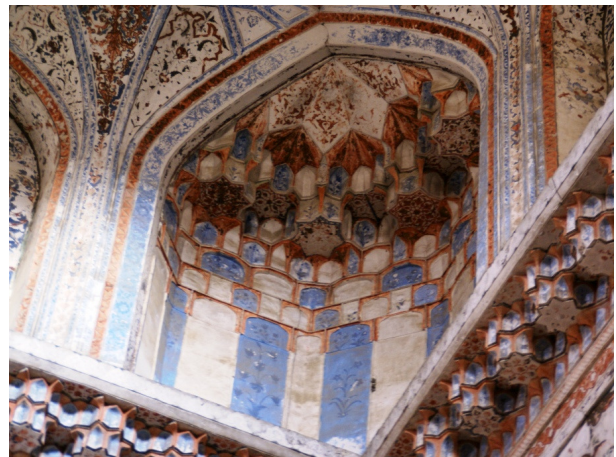
Fig.562: Bukhārā, 'Abd al-'Azīz Khān Madrasa, detail of the dome squinches, summer mosque, September 2006 Source: Author's photograph
