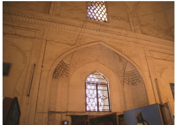
Fig.738: Bukhārā, Nādir Dīvān Beg Khānaqāh , detail of the muqarnas in an arched recess, September 2006 Source: Author's photograph
