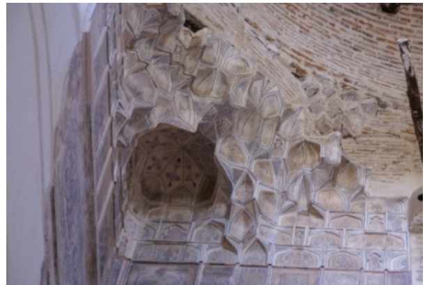
Fig.283: Shahr-i Sabz, Jahangir's tomb, detail dome squinches of the ziyarat khaneh , September 2006 Source: Author's photograph
