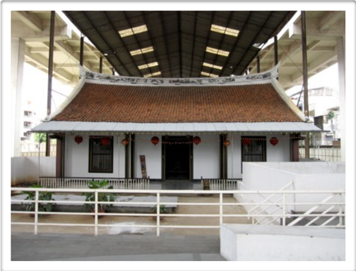
Remaining part of the grand mansion on Molenvliet of Khouw Kim An
