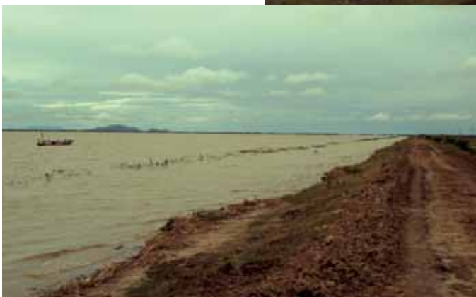
The dam and embankments of Lake Maga, built in 1979 for irrigated rice cultivation, block flooding of the Logone river and from streams of the Mandara Mountains into the southern Logone floodplain.
