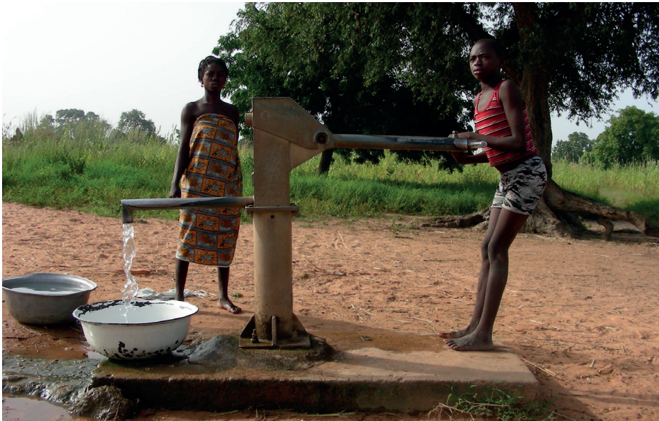
Figure 6.6 • A borehole well in the Ghanaian research area. By courtesy of L. May. Reproduced with permission.
