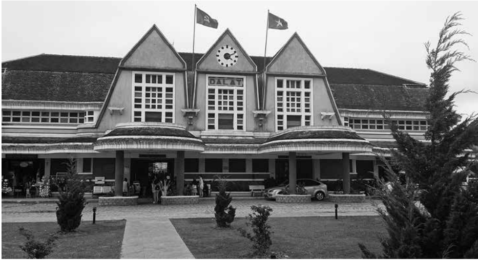
Ill. 7 The old railway station of Dalat (not used as such anymore, picture taken by author in June 2016).
