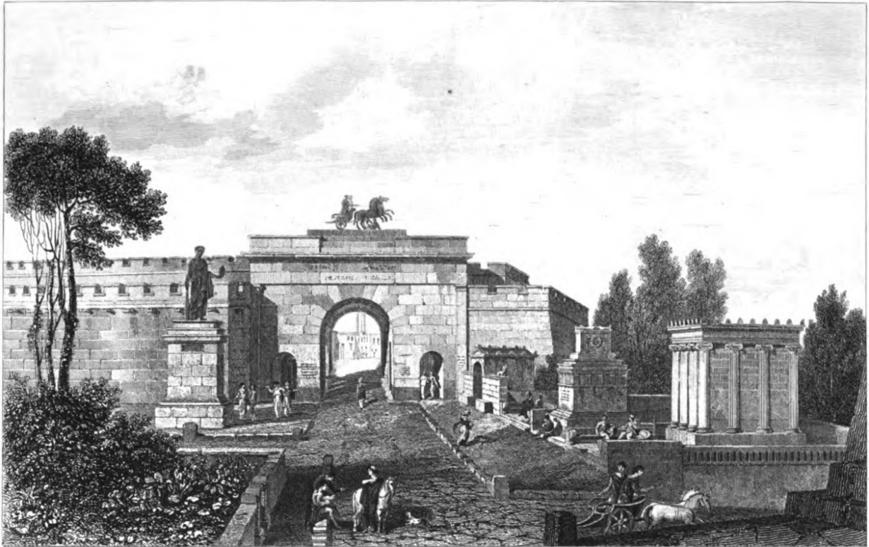
Figure 2.14 Reconstruction of one of the city gates of Pompeii (Gell 1852, pl. XIX).
