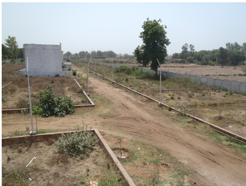
Figure 2. Housing society under construction - land converted from agricultural to non-agricultural land and divided into separate plots with low walls.
