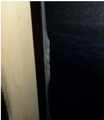
Figure 47 Detail of the damage along the left border of the first version of Lalalalight .
