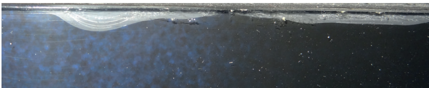
Figure 48 Detail of the damage along the upper border of the first version of Lalalalight .
