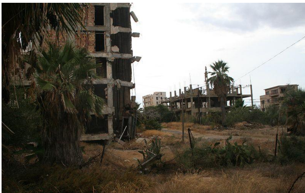
Figure 63 Photo looking into the crumbling hotels in the forbidden zone of Varosha .
