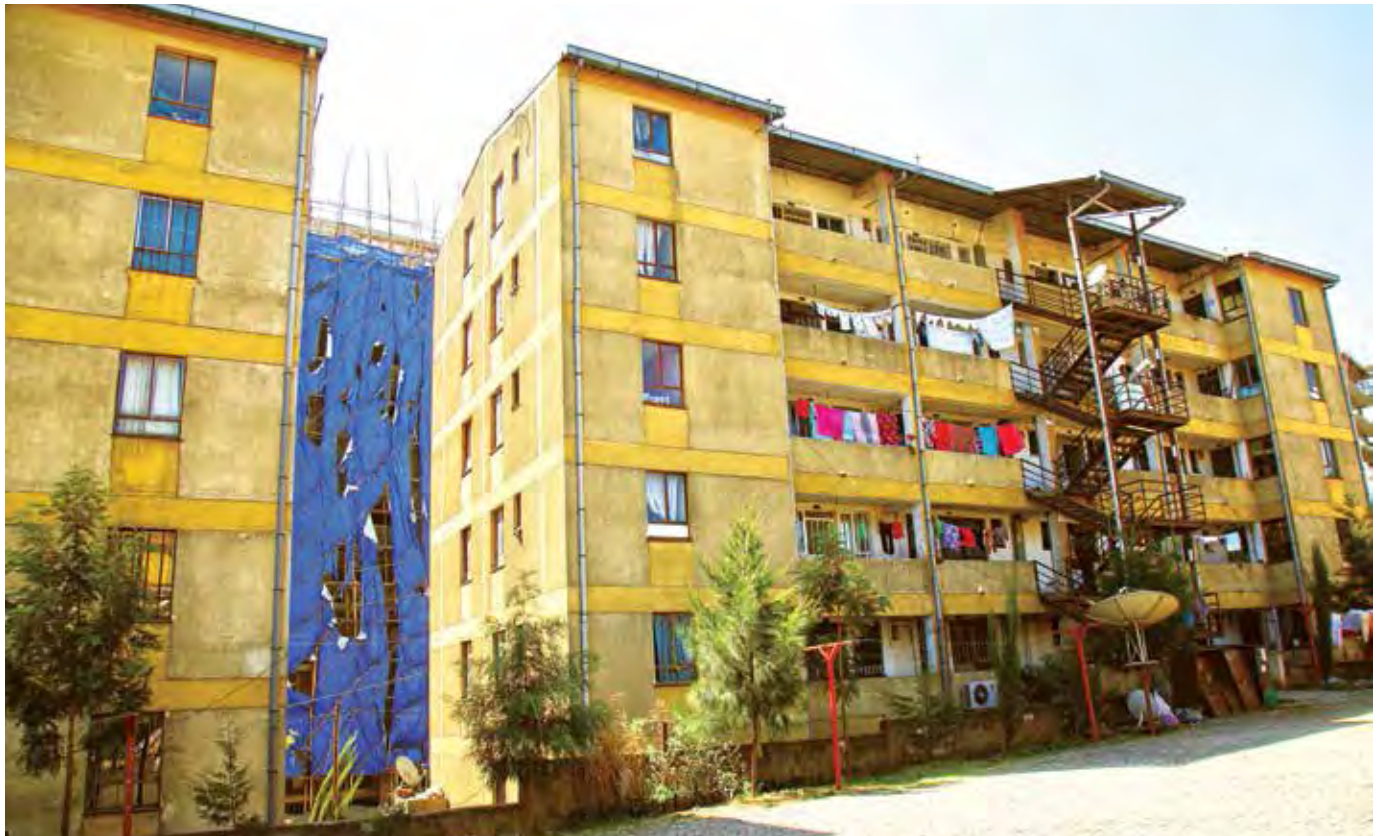
▲ Condominium housing constructed in response to housing demand. © Geo Kalev
