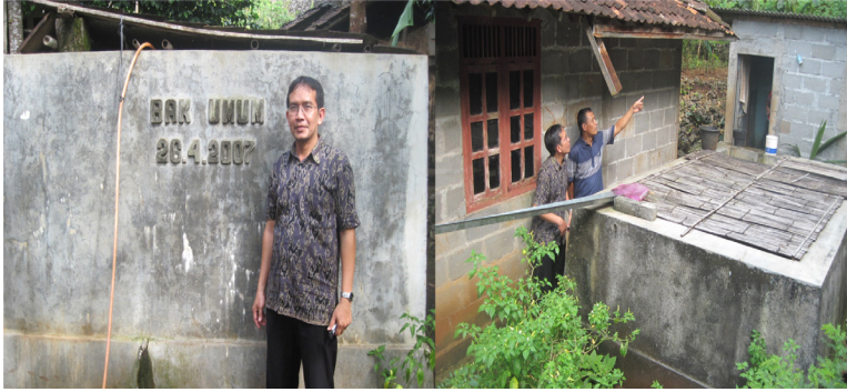
Picture 5 (left). A collective PAH capable of storing 5,000 litres of water. Source: Author's collection.
