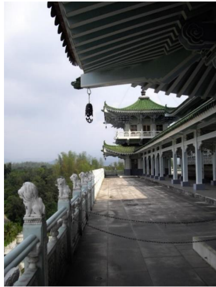
Figure 33: Hanging roofs on TOUB's roof.
